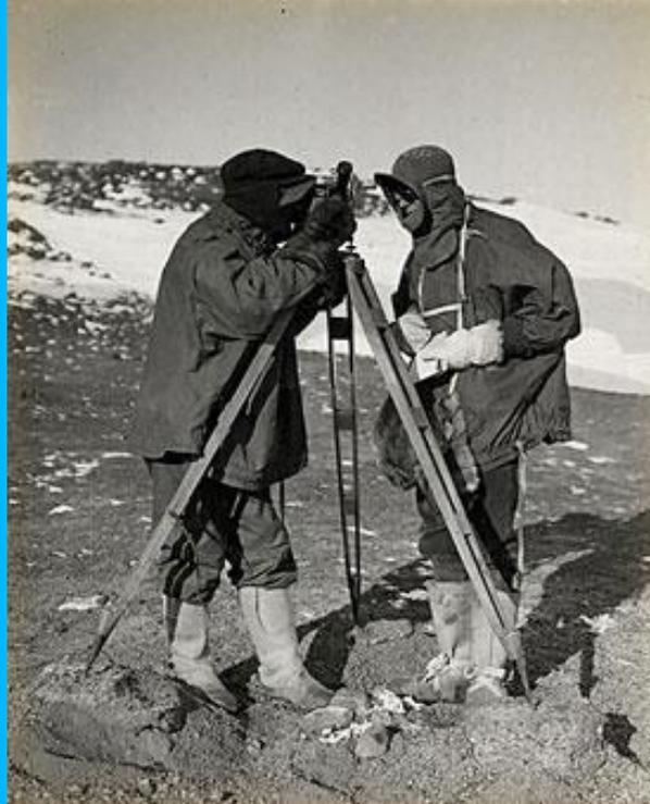
**Figure 3. Simpson and expedition member Bernard Day tracking a balloon by theodolite on “Wind Vane Hill”, a good spot for following the balloons (roughly 20m above the launch site). Photograph by Herbert Ponting. Copyright Royal Geographical Society; used with permission.**
